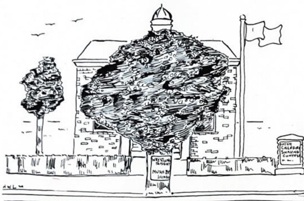
The Gymnasium taken from a difficult angle
